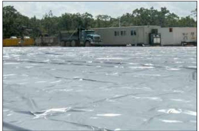
Rig-site Pad Liner
