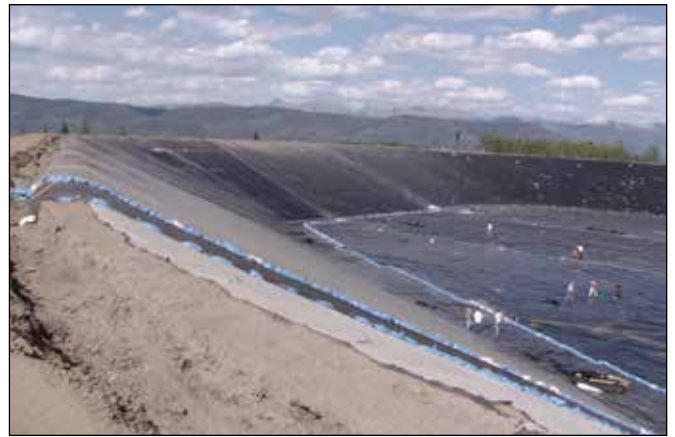
Containment Pond Liner
