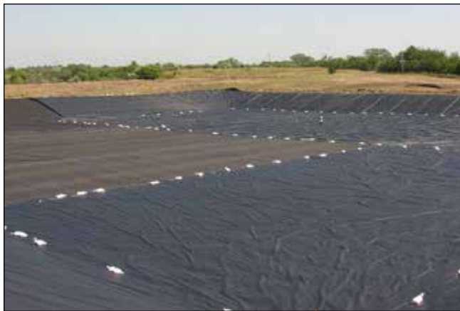
Waste Containment Liner
