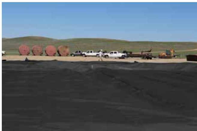
Rig-Site Pad Liner
