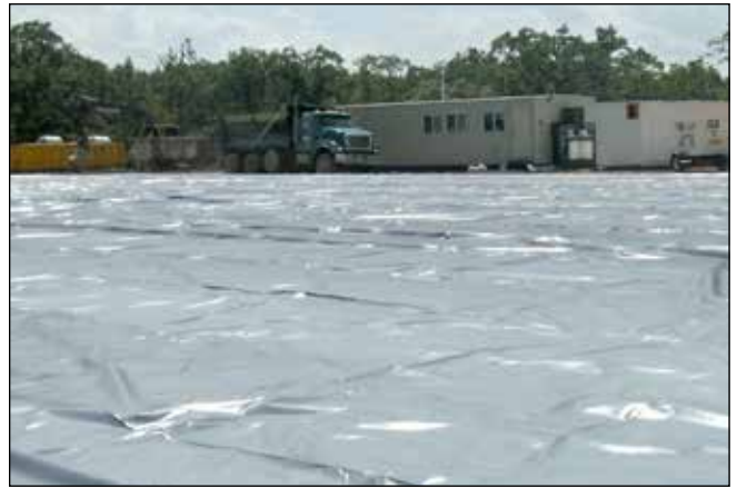
Rig-site Pad Liner
