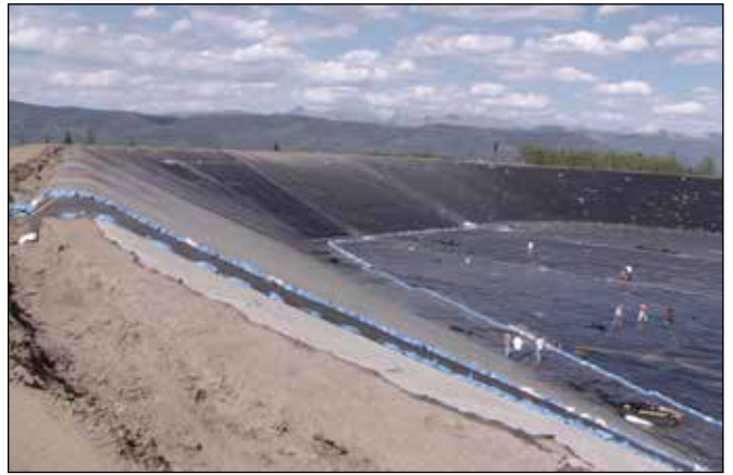
Containment Pond Liner
