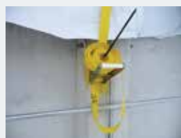
Photo 6 – Webbing tied to wall
