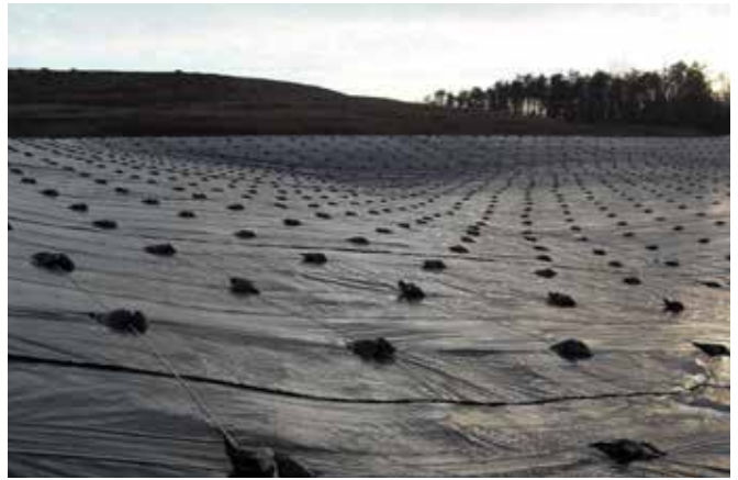
Landfill Odor Control Barrier Cover
