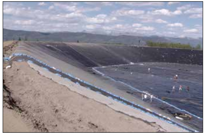
Containment Pond Liner
