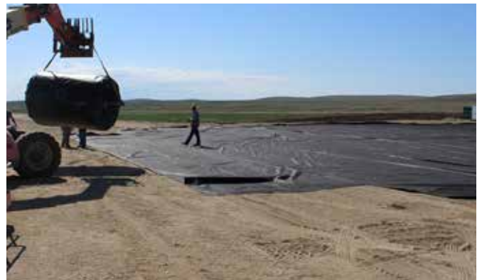
Remediation Pad Liner
