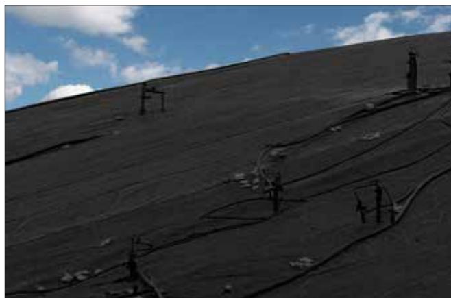
Landfill Odor Control Barrier
