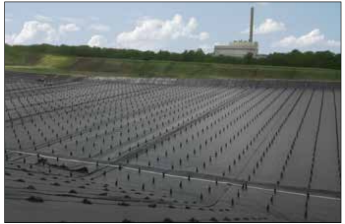
Landfill Rainshed Cover
