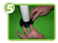
Leaving VaporBoot tape in folded position, remove entire outside release liner. Place fingers on inside of folded tape and slowly start working tape outward avoiding any folds or wrinkles in tape. Once VaporBoot tape is completely applied, press around entire section to verify seal.
