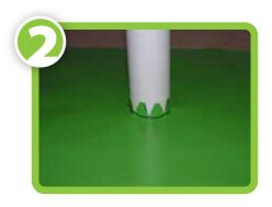
Force VaporBoot G over pipe leaving the tightly stretched cut area taut around bottom of pipe with approximately a 1/2'' of the VaporBoot G material running vertically up the pipe. (No more than a 1/2'' of stretched material is recommended to allow tape to adhere directly to pipe.)
