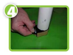
Peel off only one of the two paper release liners and apply tacky side of folded tape to the base of pipe penetration, keeping tape folded in lengthwise position. Once tape has been wrapped completely around pipe, carefully overlap ends at least 1/2" to 1" by tucking end into starting position to make a continuous seal (the very end of outside release liner will need to be peeled back about 1 1/2" to make this overlap).
