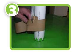
Take VaporBoot tape (supplied in VaporBoot G System package) and cut to length by measuring around pipe allowing approximately 1" extra for overlap sealing. Fold VaporBoot tape in half lengthwise forming a crease.
