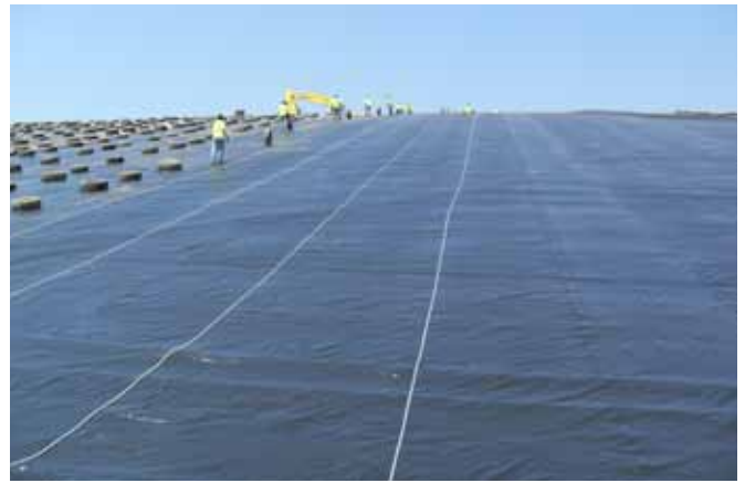
Temporary Rain Shed Cover
