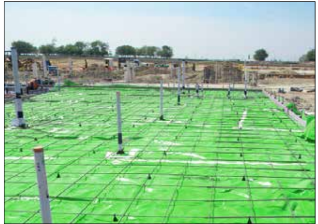
Underslab Vapor Barrier - Commercial Project
